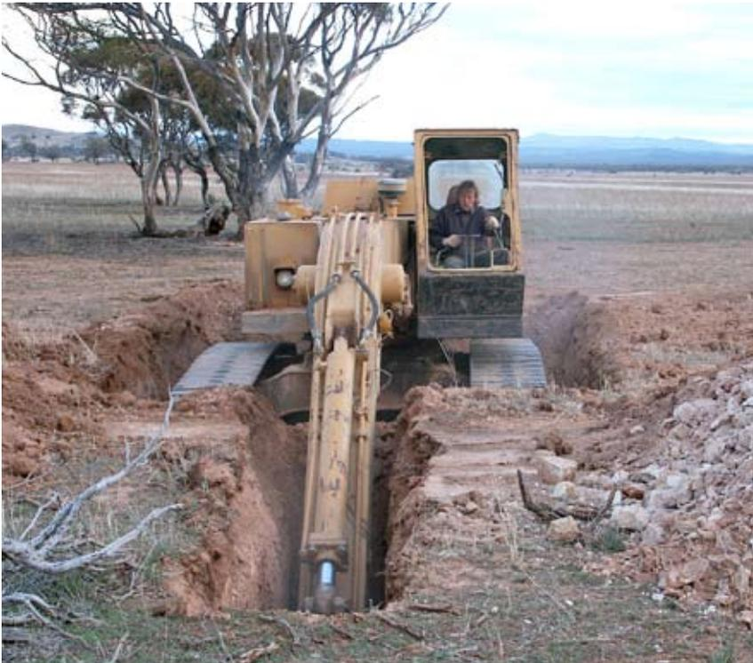
**Figure 7** Excavator "benching down" to reach a depth of seven metres at the Franklyn Target.
