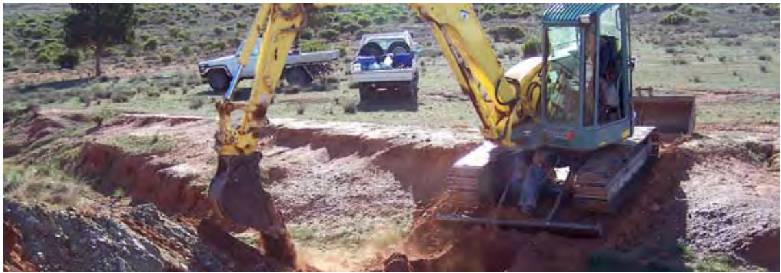
Figure 3 Recent excavator work in the Flinders Ranges
